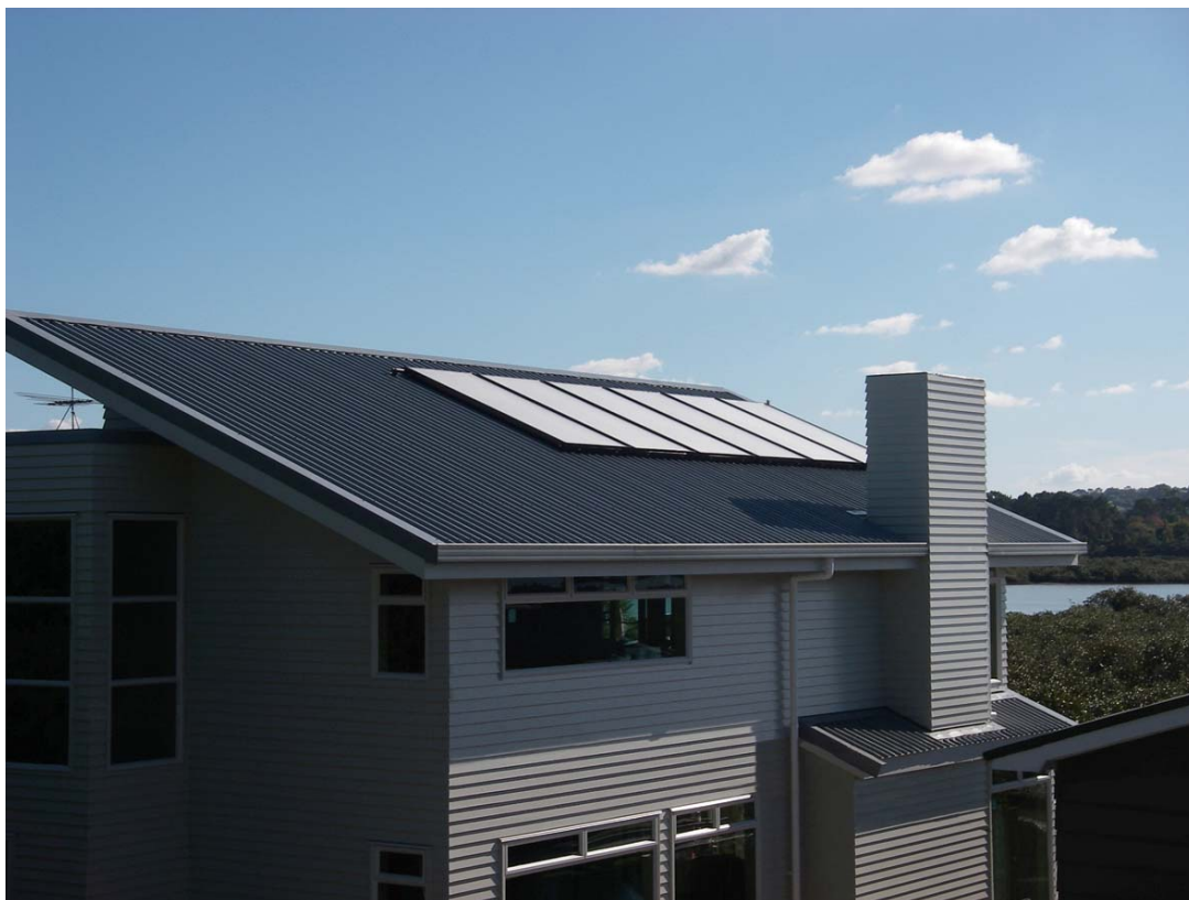
Figure 4 Large collector area installed on an indirect drainback system which manages overheating whilst maximising system performance.
